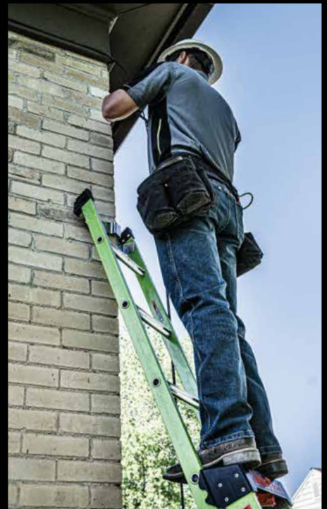
V-Bar on Outside Corner
